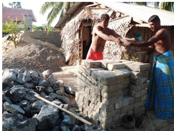
Foundations of the rice mill being constructed
